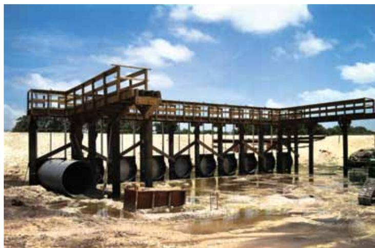
The pipe features polypropylene resin technology with a proven, dual-wall-profile design for performance and durability. The smooth interior wall offers additional strength and flow.
