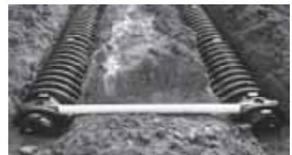
7. The “post end” has slots to accommodate zip straps in order to hang pressure-dosing pipe. Where pressure-dosing pipe is used, end caps should be prepared with a hole saw to adequately accommodate the outside diameter of the dosing pipe.
