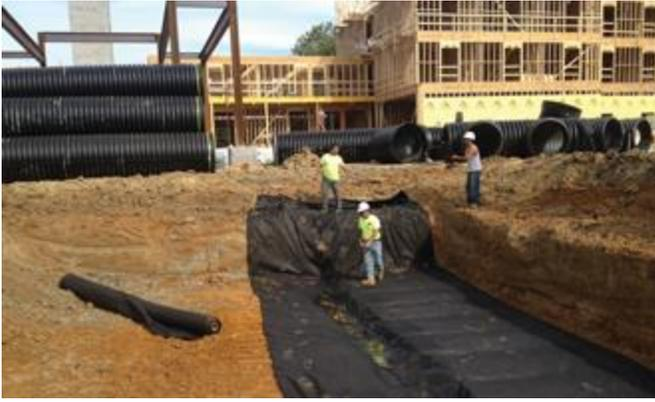
**The fabric-wrapped chambers provide for settling and filtration of sediment as stormwater rises in the Isolator Row and ultimately passes through the filter fabric.**
