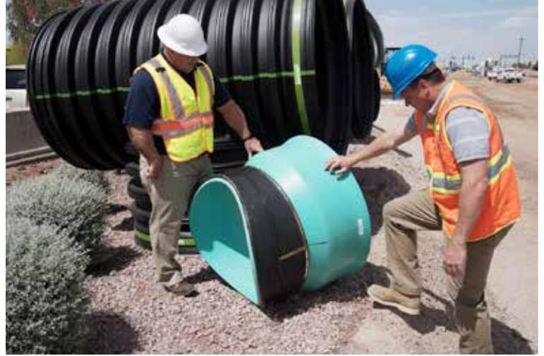
Connecting the smaller laterals to the main 54-inch lines was done using ADS Inserta Tees. They provided quick and economical watertight connections for 18-, 24-, and 30-inch HDPE pipe.
