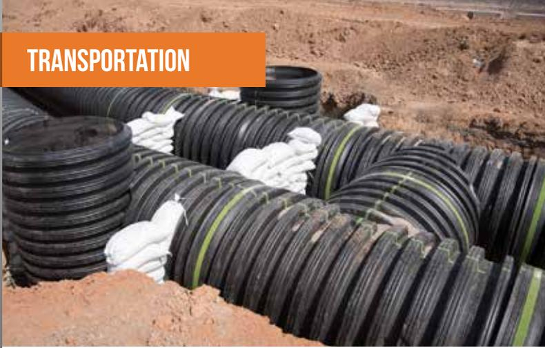
HDPE pipe provided an alternative solution to the original plan for this ADOT design-build stormwater project in Surprise, Ariz. The pipe met ADOT specifications, reduced costs, and shortened the construction schedule. Fabricated manholes were produced at the Phoenix manufacturing plant. The pipe, manholes, and other fittings were delivered to the jobsite on a just-in-time schedule.
