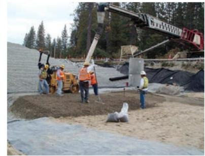
*The seismic retrofit project included rockfill buttresses hydraulic fill on the upstream and downstream sides of the concrete core wall.*
