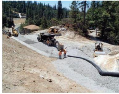
*Nearly 1,600 feet of perforated 12-inch diameter corrugated HDPE pipe was installed to allow water to infiltrate the pipe system.*
