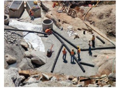
*To convey the water, 2,500 feet of 8-inch diameter, several hundred feet of 24-inch and 18-inch diameter watertight pipe was used.*
