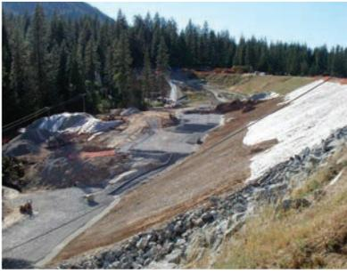
*Crane Valley Dam consists of two distinct dams separated by a rock knoll. The Main Dam is located in the main channel of the creek, and has earth fill on the upstream side of the core wall and rock fill on the downstream side.*
