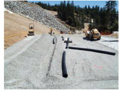
*A network of underground pipe was buried to create a toe drain that would help control any seepage from the lake.*
