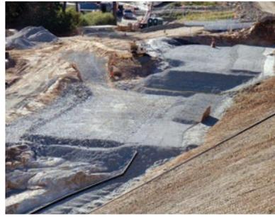
*High-density polyethylene (HDPE) pipe was used to create an underground drainage system that helps to prevent erosion of the earthen dam from seeping water. More than 4,200 feet of the pipe from ADS was used on the dry side of the two dams to pull groundwater away from the bottom of the structures.*
