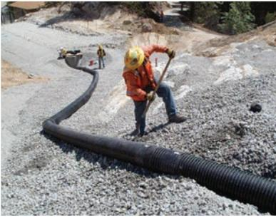
*ADS N-12® soil tight perforated and watertight corrugated HDPE pipe was used to create the toe drain and to provide drainage under other areas of the dam.*
