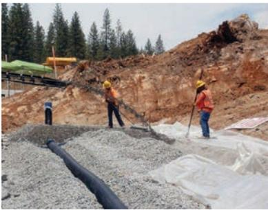
*The dam modification used an additional 253,000 cubic yards of rock fill to selected areas on the upstream and downstream faces of the dam.*
