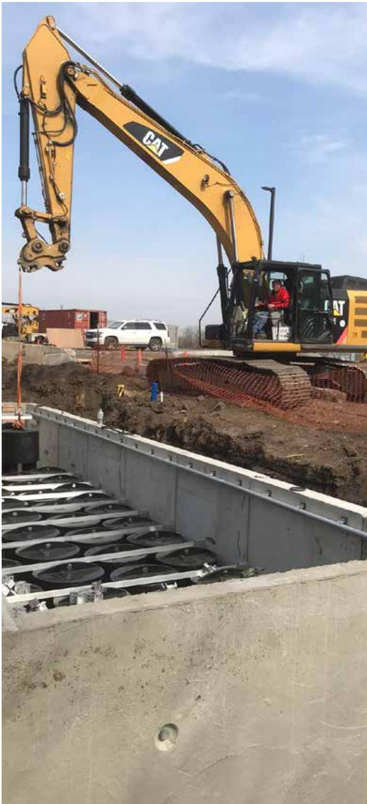
An ADS BayFilter is lowered into place in one of the two concrete vaults at the old Harrison Avenue landfill in Kearny, N.J. Each BayFilter unit can trap 80 percent of total suspended solids, meeting New Jersey's requirements.
