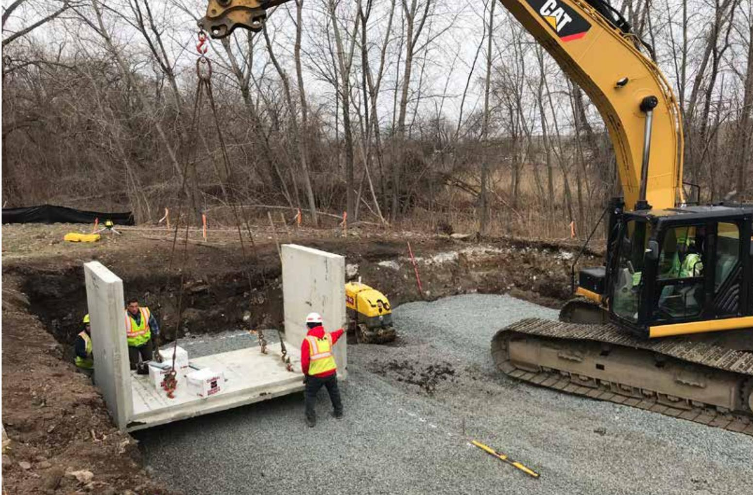
Two concrete vaults were designed and delivered in pieces that could be put in place using an excavator so the contractor would not have to add a crane to the heavy equipment list.
