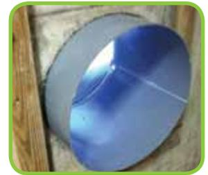
Figure 17: End Wall Connection with Adapter
