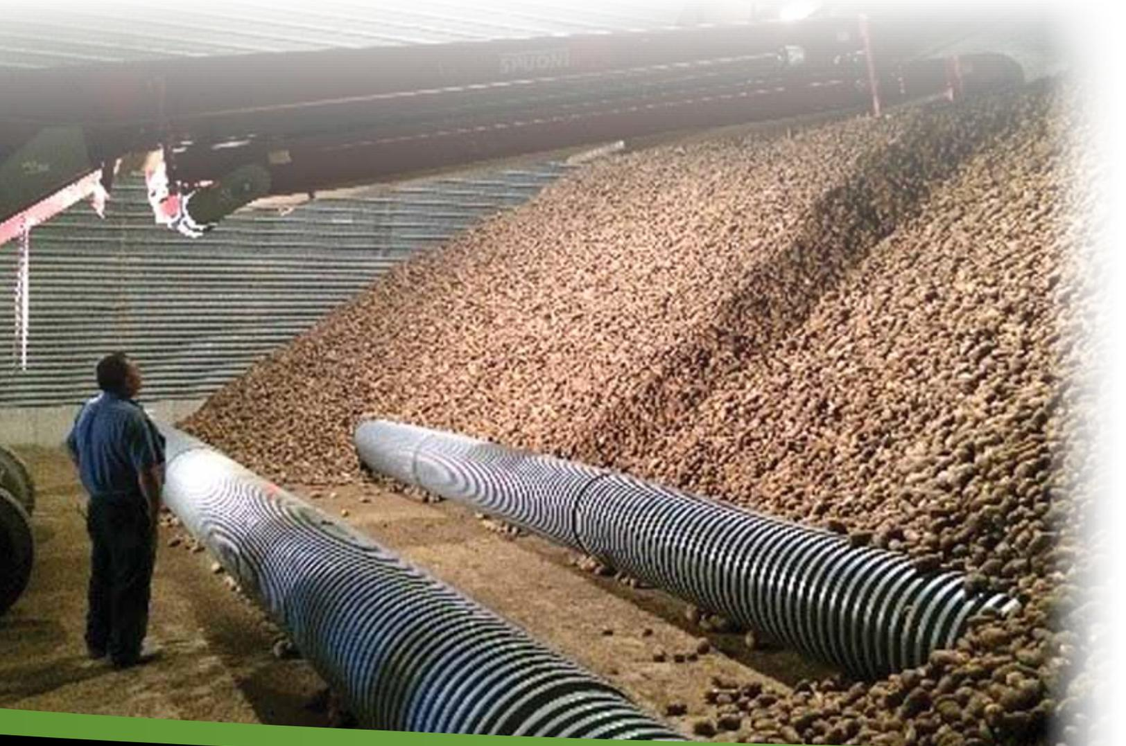
are provided where each pipe run will connect in order to aerate the potato pile. The outside diameter of ADS pipe is comparable to other corrugated pipe products and a reasonably snug fit is provided by simply butting/inserting the pipe into the existing hole (Figure 16). Alternatively, an adapter (thin-walled tube welded to ADS pipe) can be provided for installations where a smaller diameter is desired or if the pipe needs to protrude further through the wall (Figure 17).
