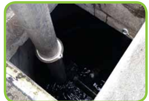
Jet Vactoring Through Access Hatch
