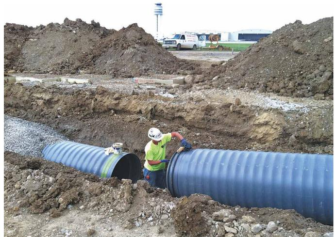
Lightweight and easily maneuverable ADS SaniTite HP polypropylene pipe helped increase efficiency in installing a new stormwater drainage line at Port Columbus International Airport.
