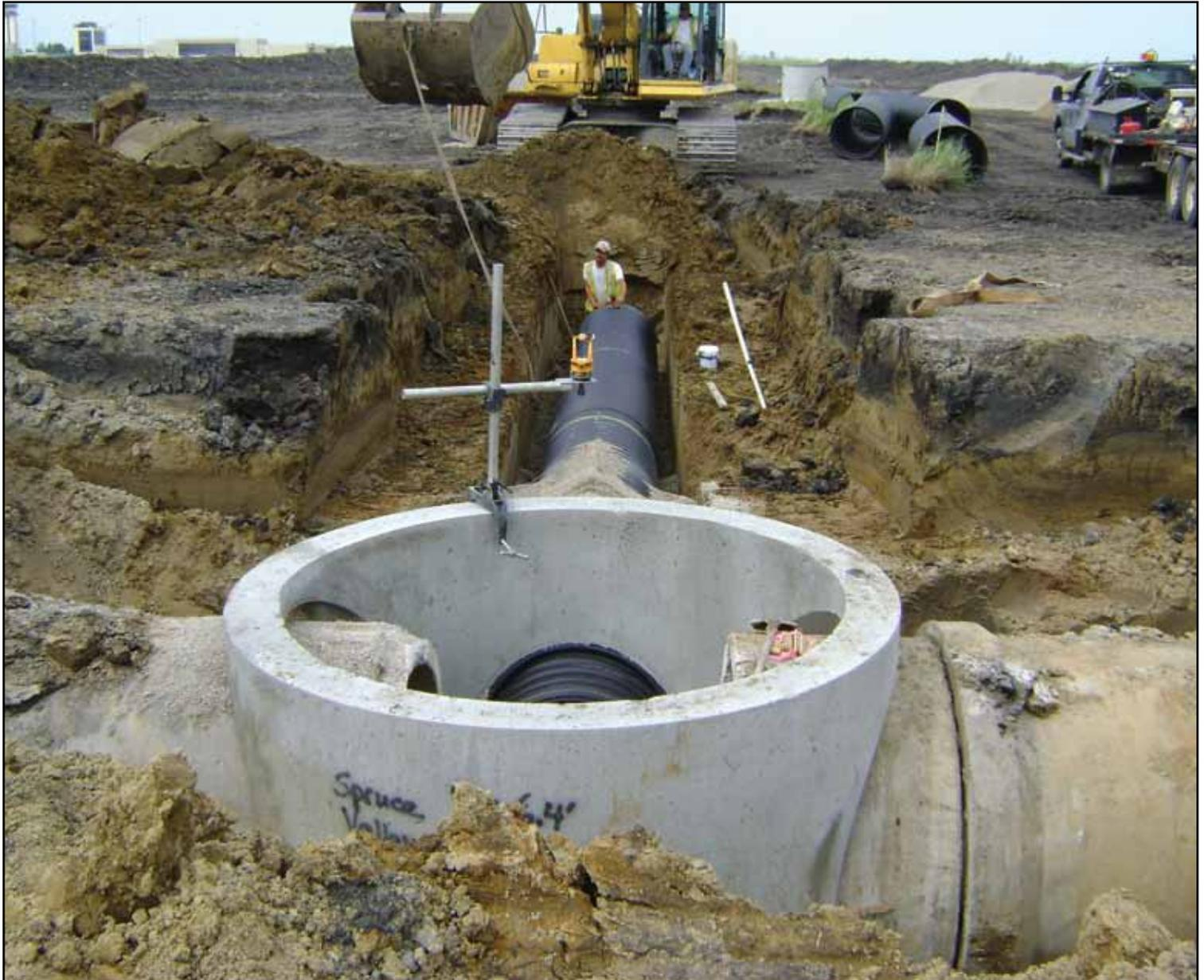
**More than three miles of HDPE pipe from Advanced Drainage Systems was used to provide a solution to a high water table at the Grand Forks International Airport.**
