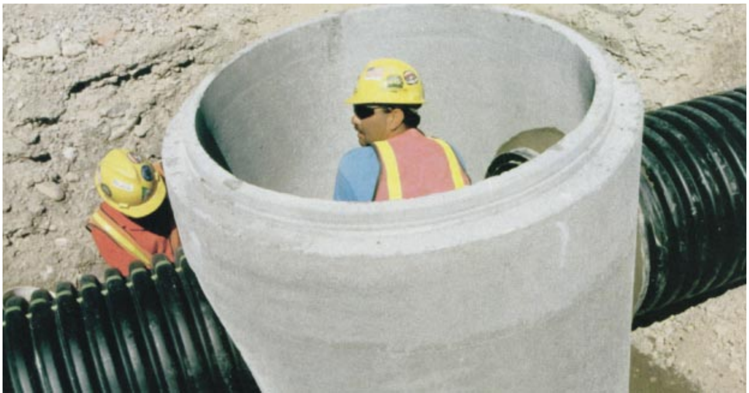
The pipe has a neoprene gasket on the outer rim of the spigot end of the pipe to meet all soil-tight applications.
