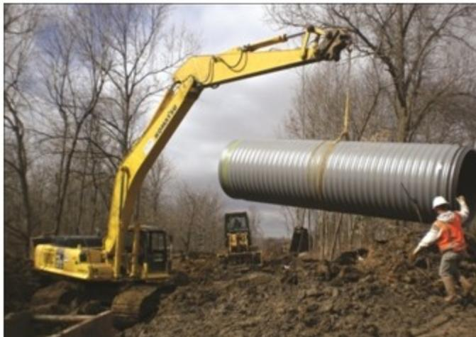
**MOBERLY, MO - Located in the middle of Missouri about equal distance from Kansas City and St. Louis, the City of Moberly replaced an aging sewer line with 60-inch diameter pipe from ADS.**
