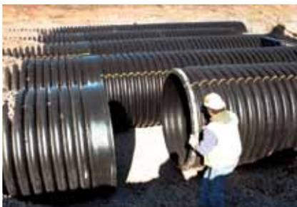
More than 2,500 ft of 60-in.-diameter corrugated HDPE pipe was used to construct an underground retention system capable of storing 85,000 cu ft of water.
