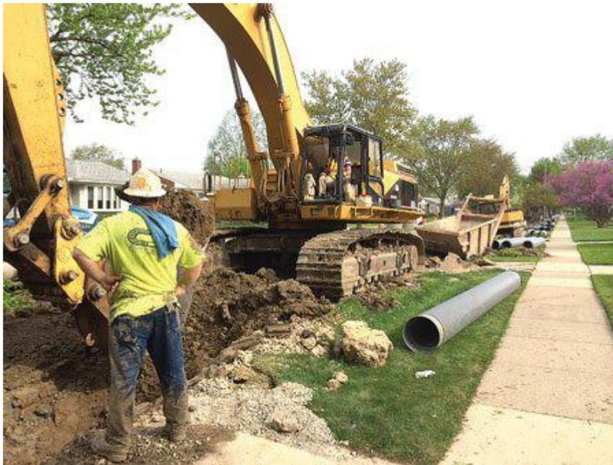
The project used some 900 linear feet of 12-inch and 1,700 linear feet of 15-inch diameter SaniTite HP pipe.
