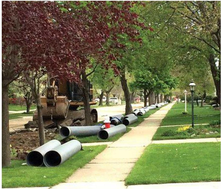
**To prevent recurring backups of sewage into the basements of Southgate residents, engineers designed a relief sewer line using polypropylene pipe.**
