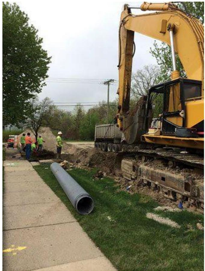
**The pipe was installed using cut-and-cover at depths ranging from 12 to 22 feet.**
