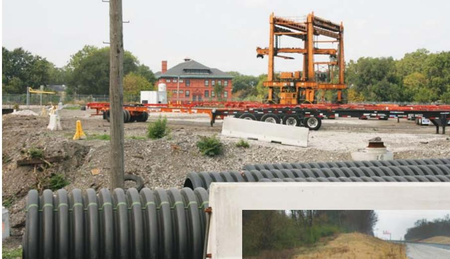
**Left:** Large-diameter corrugated HDPE pipe waiting to be installed at a depth of 13 ft.
