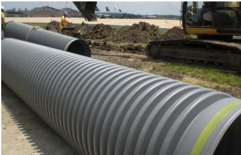
*Advanced Drainage Systems' corrugated polypropylene pipe was selected for the drainage project.*
