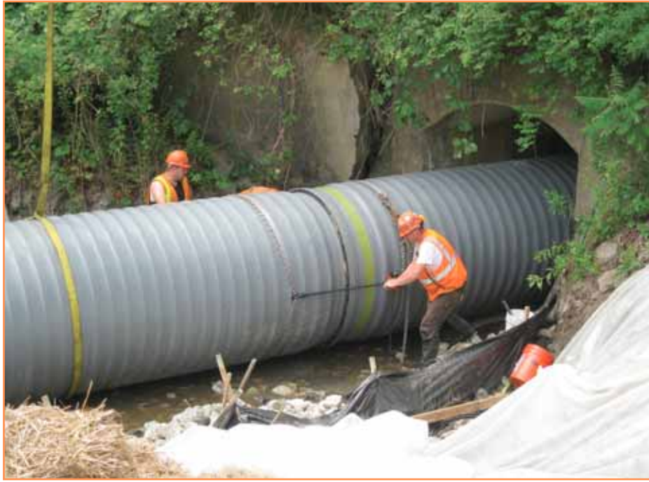
Contractor easily assembles the field joint together with ratchet straps.
