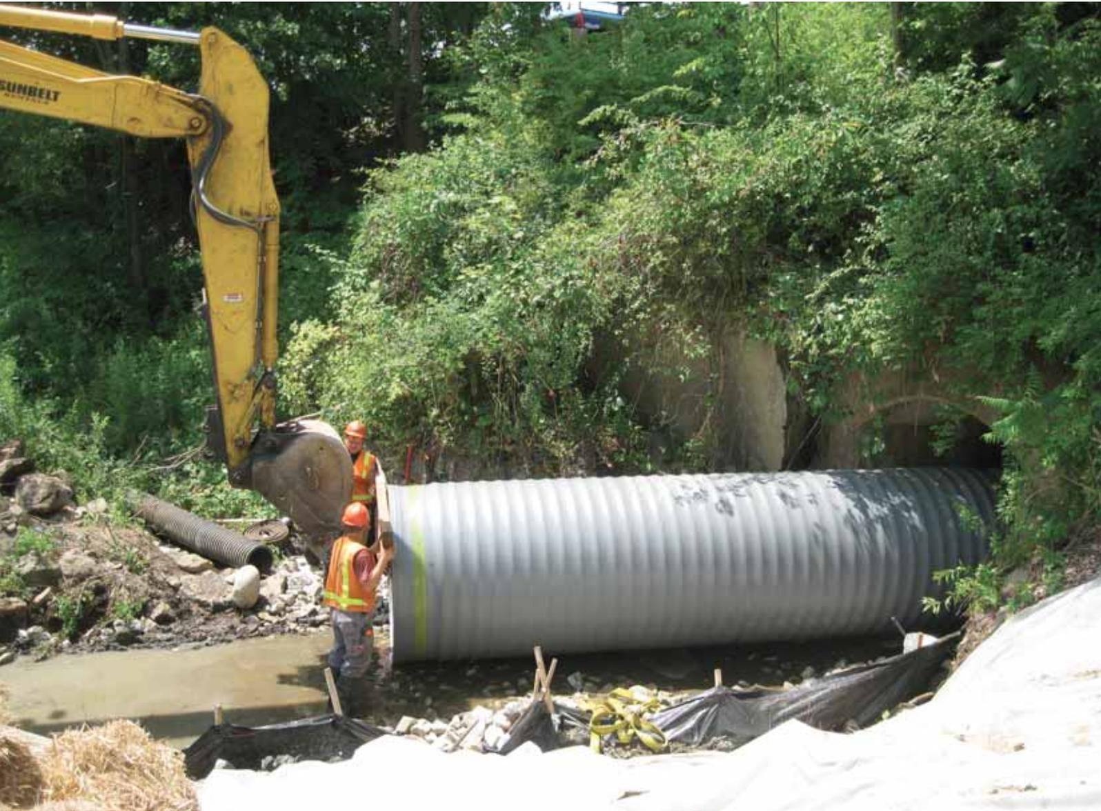
**A 20-foot section of SaniTite® HP pipe being nudged into the culvert. It took the crew just hours to slipline the entire 200 feet of the culvert.**
