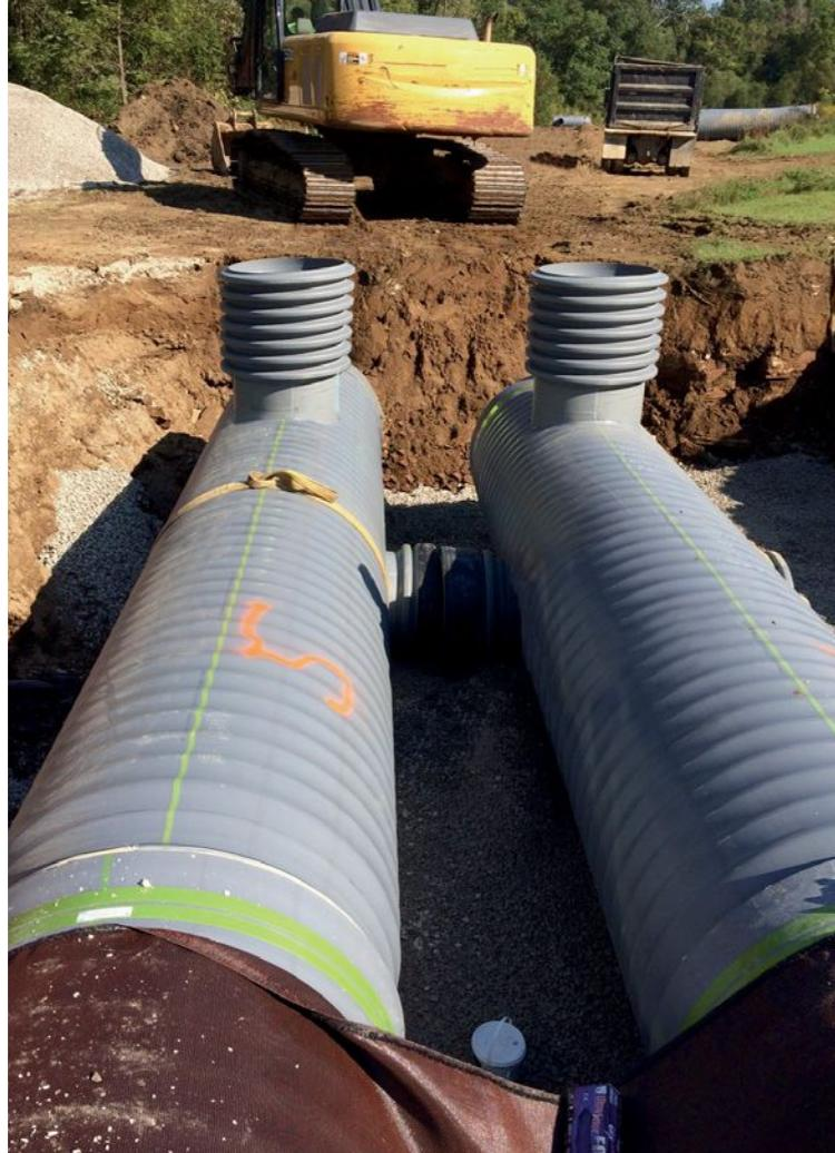
The new pipe system temporarily stores wet weather volumes upstream of the lift station. The water will then flow from the pipes to the lift station and be pumped to the treatment plant.
