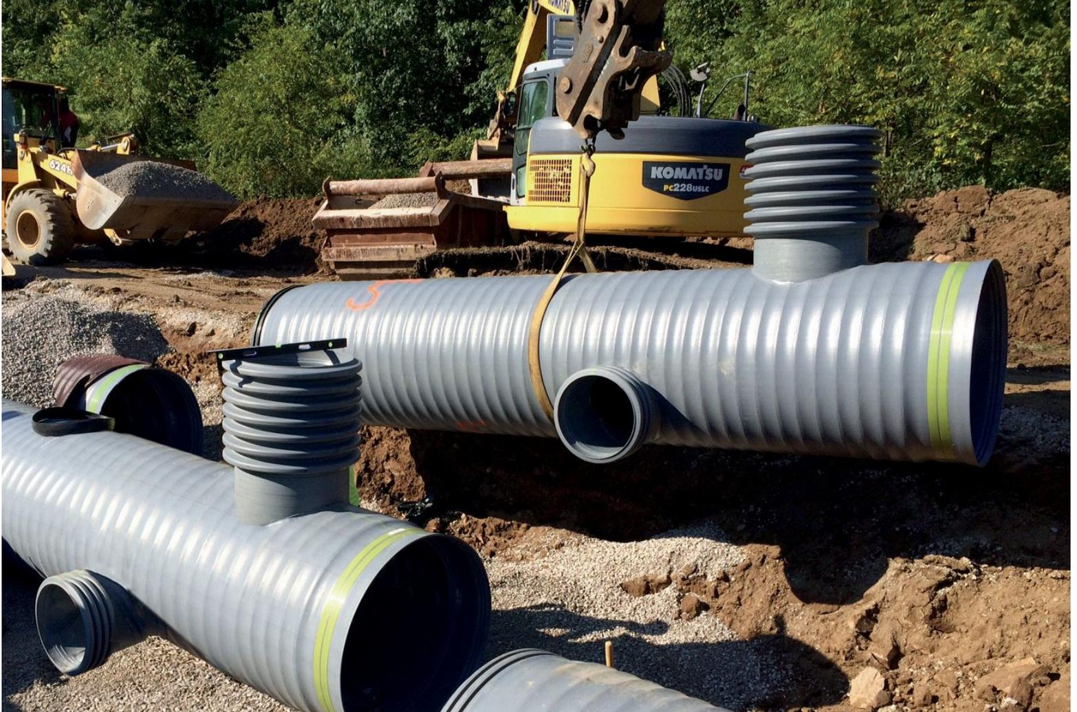
A total of 1,600 feet of 48-inch-diameter ADS SaniTite HP polypropylene pipe with eight risers was used for the detention pipe system. Cover ranges from three to four feet.
