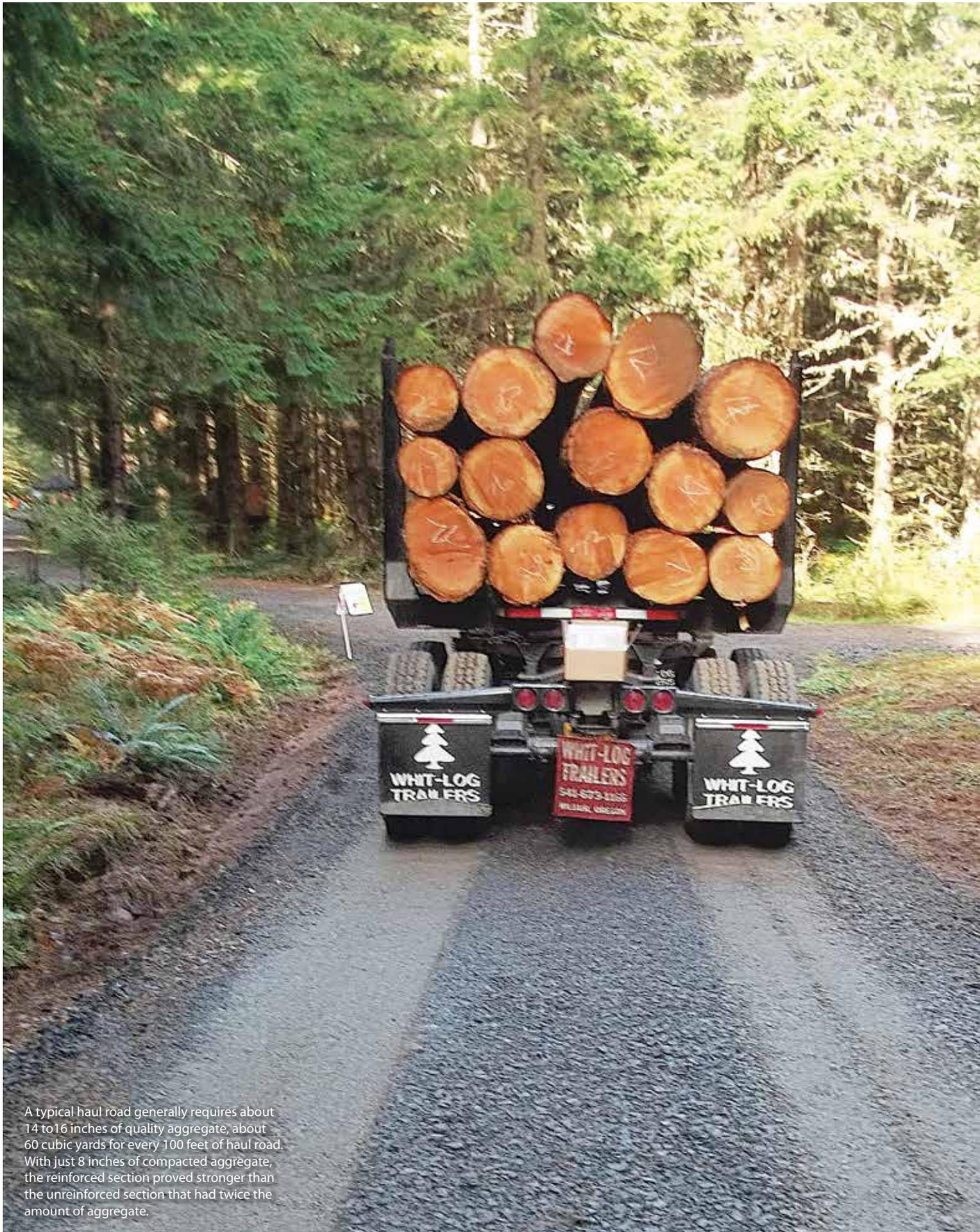
A typical haul road generally requires about 14 to 16 inches of quality aggregate, about 60 cubic yards for every 100 feet of haul road. With just 8 inches of compacted aggregate, the reinforced section proved stronger than the unreinforced section that had twice the amount of aggregate.
