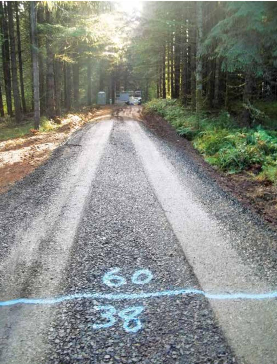
An aggregate haul road was constructed to demonstrate the difference of an unreinforced section vs. a section reinforced with geogrid.
