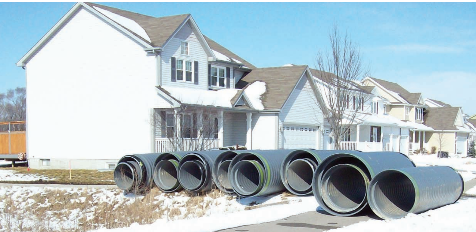
Figure 2: Grimes Pipe 6 Staging
