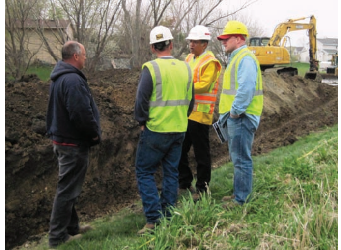
Figure 4: Installing the New Sanitary Sewer Line
