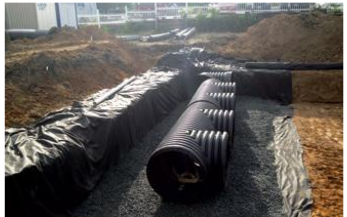
The open-bottom chambers and perforated sidewalls allow stormwater to flow both vertically and horizontally out of the chambers.
