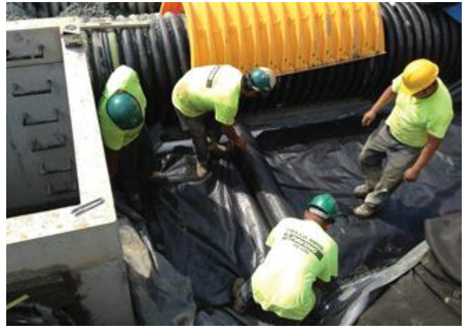
A woven geotextile fabric filters stormwater, provides a durable surface for maintenance, and prevents scour of underlying stone. A non-woven fabric provides a filter media for flows passing through the perforations in the sidewall of the chamber.
