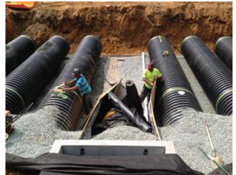
The Isolator Row is a series of StormTech chambers surrounded with filter fabric and connected to a closely located manhole for easy access.
