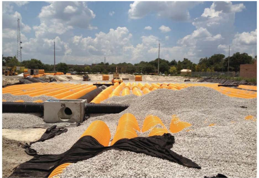
The Isolator Row (center) is a series of StormTech chambers wrapped in filter fabric and connected to a manhole for easy access.
