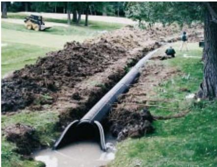
**ADS N-12® smooth interior pipe** provides excellent flow and durability for rapid outlet and transfer of collected storm water. Diameters from 4" through 48", perforated or non-perforated.
