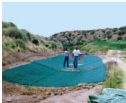
ADS offers a complete line of geotextile construction fabrics, silt fencing, geogrids, and erosion control mats for soil stabilization, reinforcement, filtration, separation, and sub-surface drainage.
