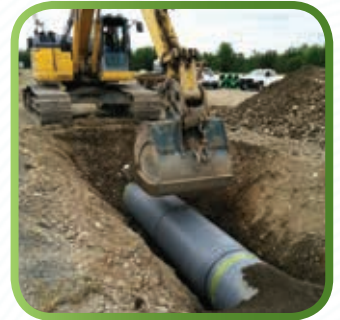
WSDOT Project: Mellen Junction, Chehalis
