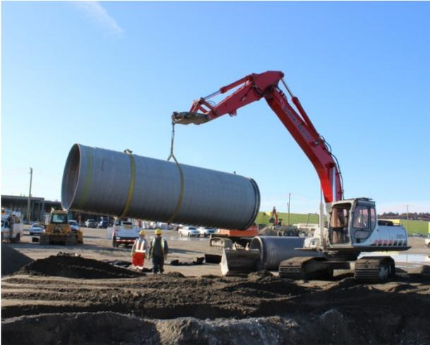
Delivered from the recently opened ADS distribution yard in Abbotsford, a 6-meter (20-foot) long section of large diameter SaniTite HP pipe is moved into place for a nearby mega-mall project.
