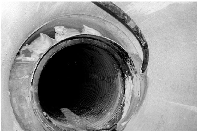
It is common for aging metal culverts to have deteriorated or completely destroyed inverts. This allows the fluid carried through the culvert to create void space under the pipe, creating an undesired condition. The grout material will help plug and fill any fractures or holes in the existing culvert along with structurally stabilizing the system from thermal effects, hydrostatic pressure, point loads, and function as a water barrier.
