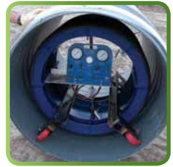
Joint Isolation Test
