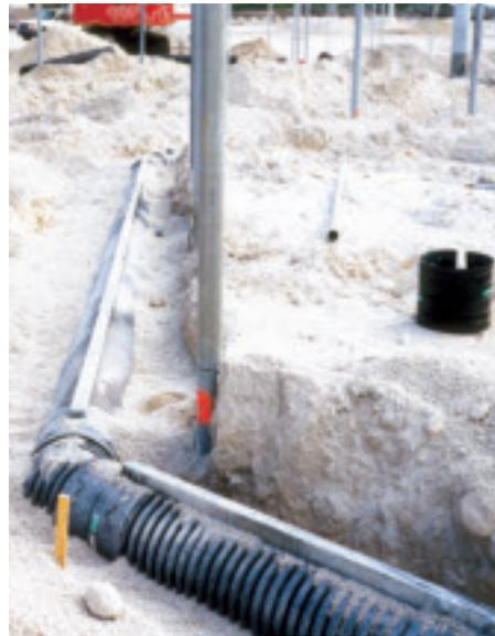
A total of 1,540 ft. of Duraslot 12" drain with a 2.5" slot height were installed.
