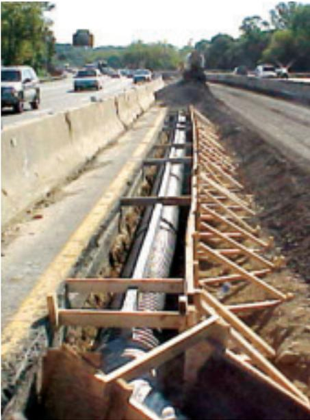
More than 11,000 ft. of 15" Duraslot drains were installed on the project. Contractors estimated that installation time was reduced by at least 20%, saving not only project costs, but also the time traffic would be backed up due to crossover construction.
