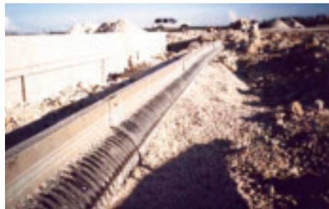
Smooth inner wall N-12 pipe resists chemical attack and provides superior hydraulic flow compared to corrugated steel pipe.
